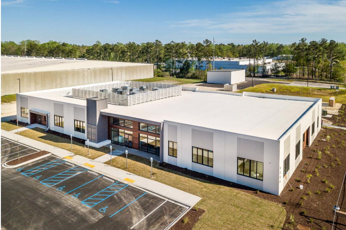
Rogers & Brown's New State of the Art Headquarters Building- Ladson, SC
